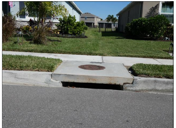
Stormwater Drainage Curb Inlet
