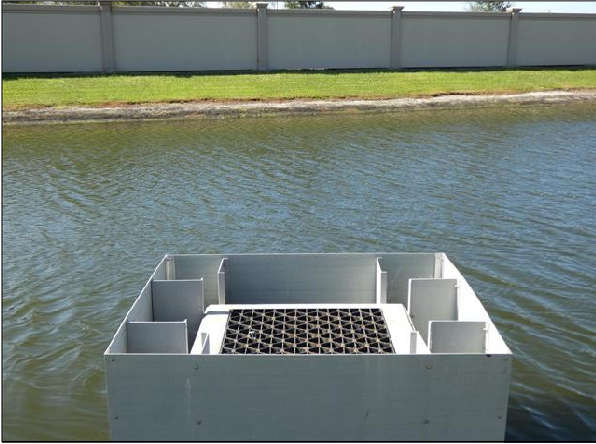
Stormwater Drainage Control Structure
